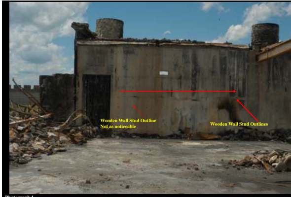
Photograph 4 This photograph is looking west from inside of the residence. The library turret would have been located to the left of the doorway in the concrete wall. The concrete wall separates the Library, Dining Room and Kitchen from the garage. The red arrow indicates the direction of fire movement.
