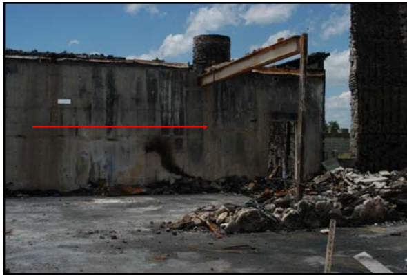
Photograph 5 Same wall as Photograph 3, looking more to the right. The Kitchen Turret is located at the right side of the photograph. The red arrow, indicates the direction of fire movement.
